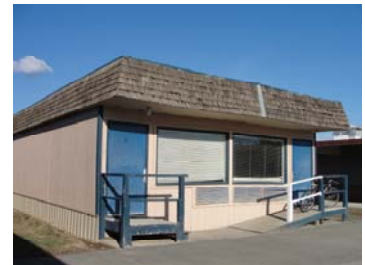
Asbestos and lead survey at a school
