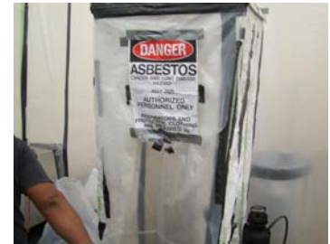
Asbestos abatement oversight
