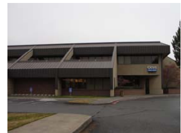
Asbestos survey at a credit union
