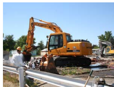
Lead (Pb) air testing during demolition
